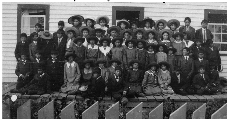
All Saints IRS, Lac la Ronge, Saskatchewan was supported by Kootenay Diocese.
