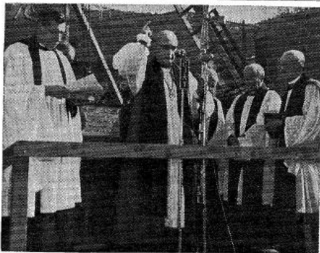
Laying of the foundation stone of the new St. Andrew's Church, Trail, by the Right Reverend W. F. Barfoot, former Primate of Canada, assisted by: Left to right—Reverend J. Rogers, Right Reverend Mr. Barfoot, Reverend W. Edington, Archdeacon B. A. Resker, and Archdeacon F. H. Graham.
