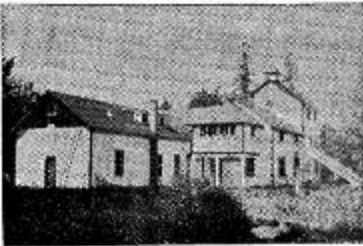
Vernon Preparatory School (Old School)
